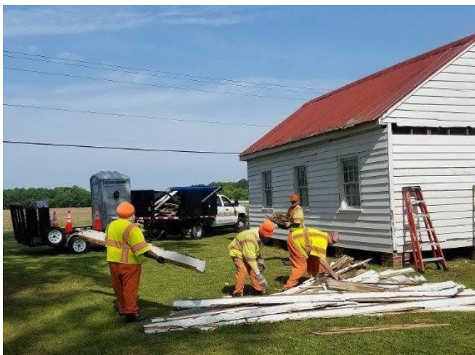
Workforce inmates working on the Pleasant Ridge Elementary School renovation.
